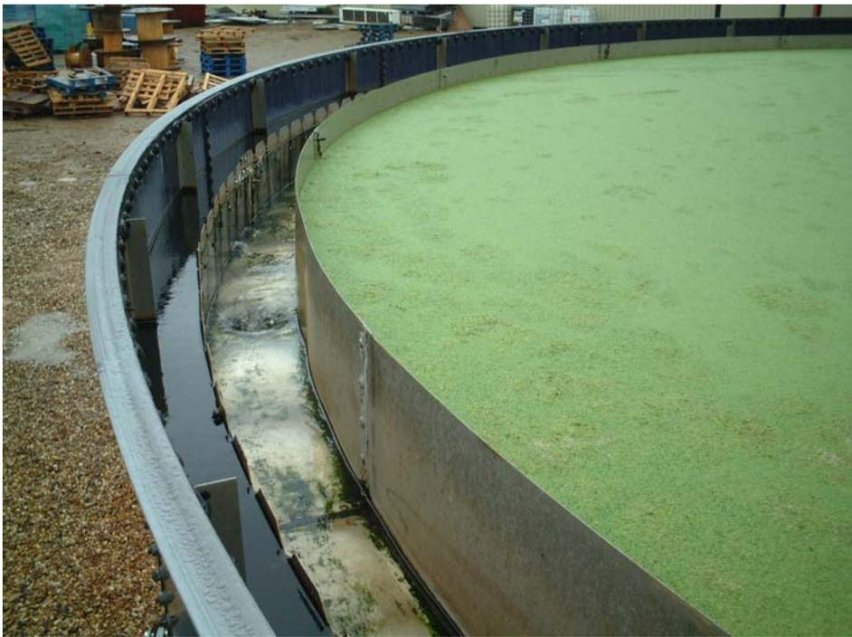
**Figure 2 Stainless Steel Weir in Tank**
