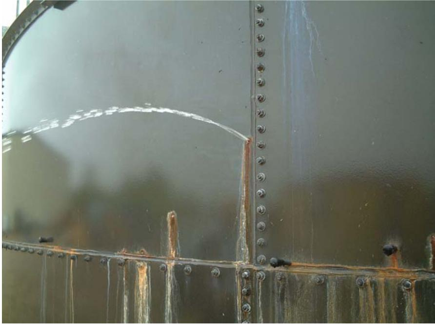
**Figure 3 Result of Inadequate Internal CP**
